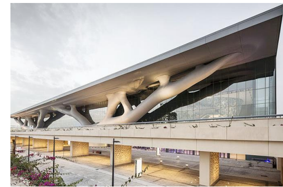
Fig. 16 Building structure topology optimization [12]
